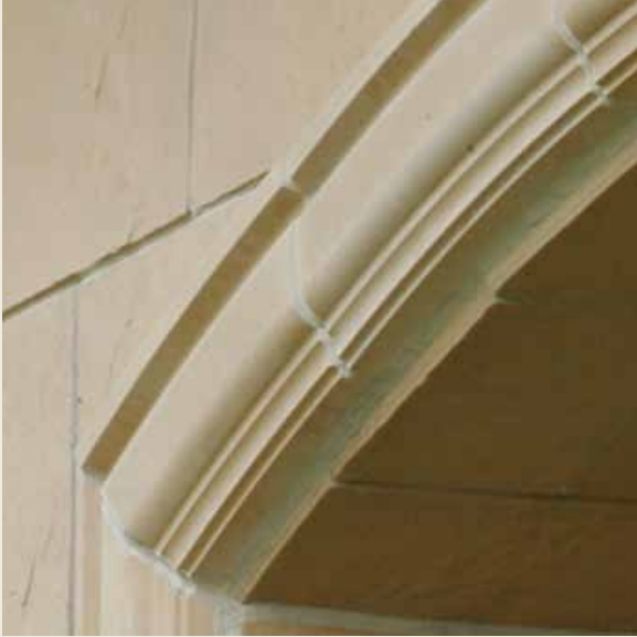
ABOVE: Molding #1 creates this graceful arch with slate tiles.
